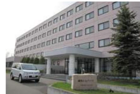
The dormitory at the Tokachi Proving Ground provided to disaster victims free of charge
